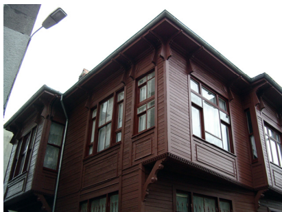
House repaired by Turkish Timber Assoc.
