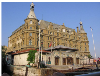
Haydarpaşa train station
