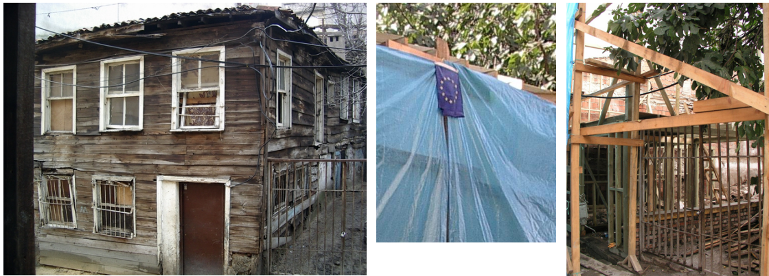
One of the two demolitions carried out by EU funded project
