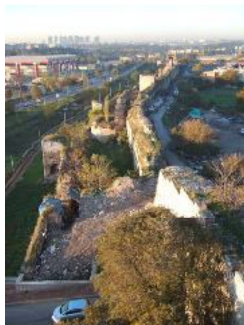
Above right: tower after rubble has been bulldozed over part of the collapsed structure of the tower, to create parking between the inner and outer walls, 2007
