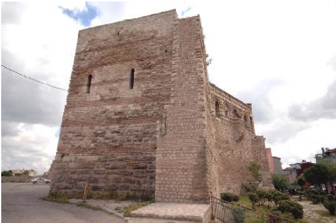
Above: junction of the Theodosian Land Walls and Tekfur Saray. Work carried out since the 2006 mission has falsified the evidence of the structure by creating a new, false, wall end to a collapsed section of the wall, in which the brick banding is carried in the form of brick stretchers completely across the stone core.
